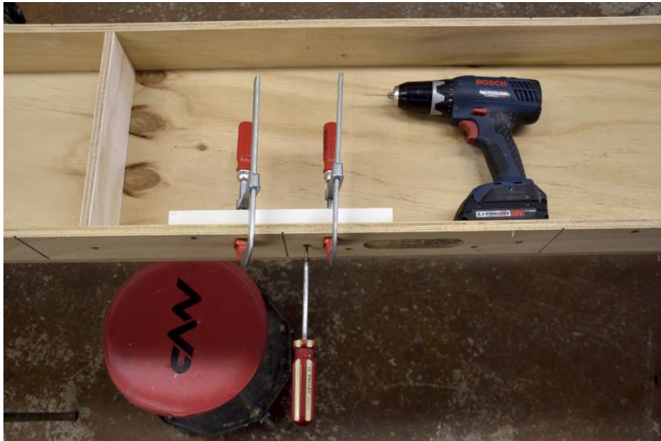
Photo 4. Installation of Internal Brace
