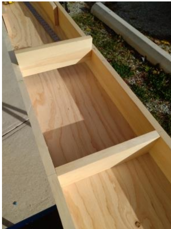
Photo 3. Install Gussets Inside Box
